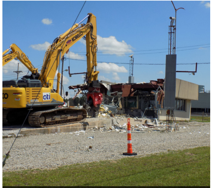
The 720-F Central Alarm Station that was successfully demolished down to a slab.
